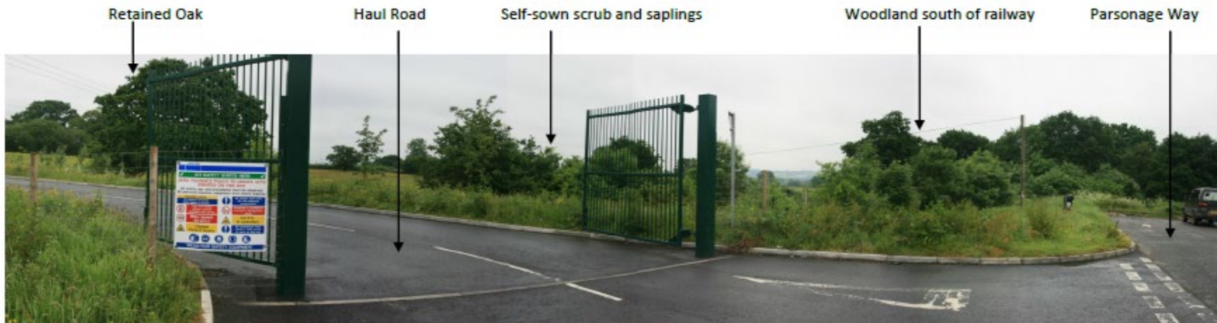
PANORAMA A - from junction of new Haul Road with Parsonage Way, looking east
